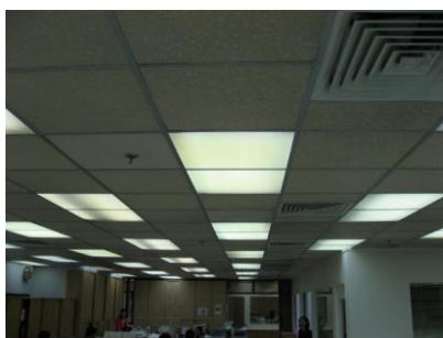
Before the installation of Nanoflex™
