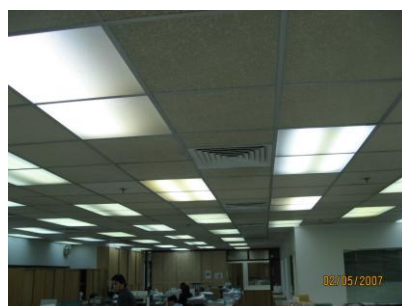
After the installation of Nanoflex™
