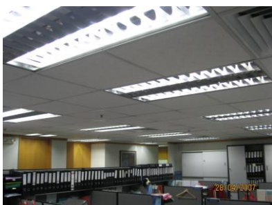
After the installation of Nanoflex™
