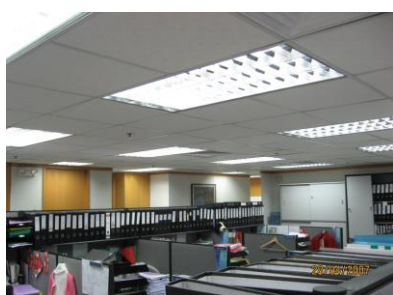
Before the installation of Nanoflex™
