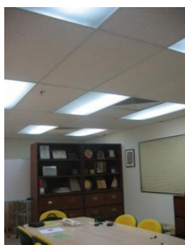
After the installation of Nanoflex™
